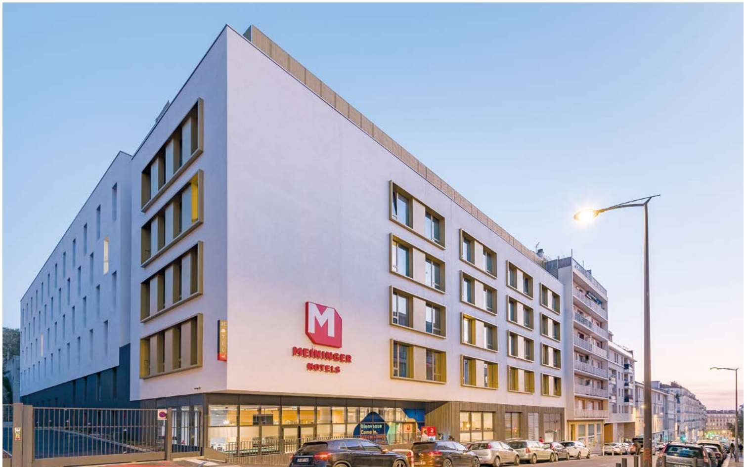
25-27, rue Forbin - Marseille (13) Acquisition 2020
