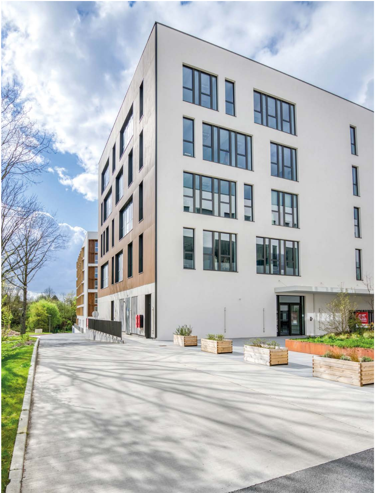
5, avenue Augustin Louis Cauchy - Nantes (44) Acquisition 2019
